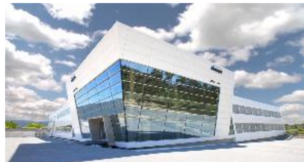
Figure 58 - Aimen Laser Centre at Porriño (Spain).
