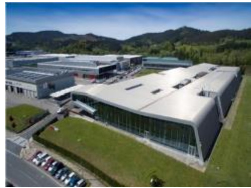
Figure 60 - The AIC in Amorebieta, Spain.
